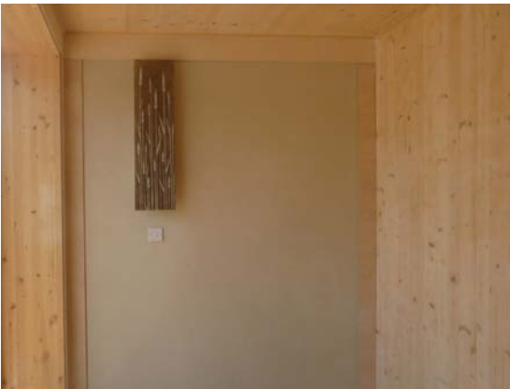
ModCell® traditional showing light switch installed in lime render
