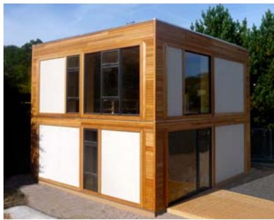
Photo supplied by Modcell
